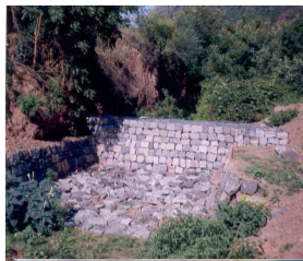
Gabion Structure near Kalimangalam Village
