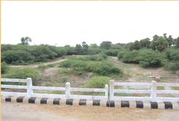
GRIDHUMAL RIVER NEAR KARUVAKKUDI BRIDGE- D/S
