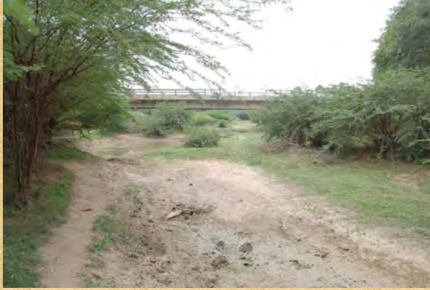
GRIDHUMAL RIVER NEAR KARUVAKKUDI BRIDGE- U/S
