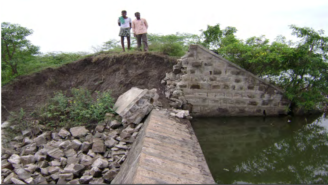
M.JEGAVEERAPURAM TANK—DAMAGED SLUICE
